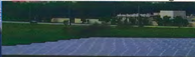
Apra Substation Site
